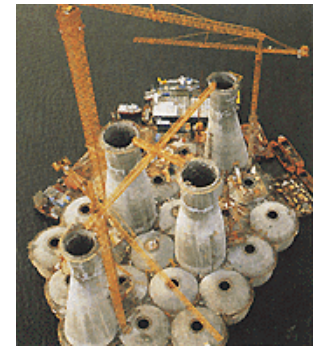
The sinking of the Sleipner A offshore platform (inaccurate finite element approximation)
